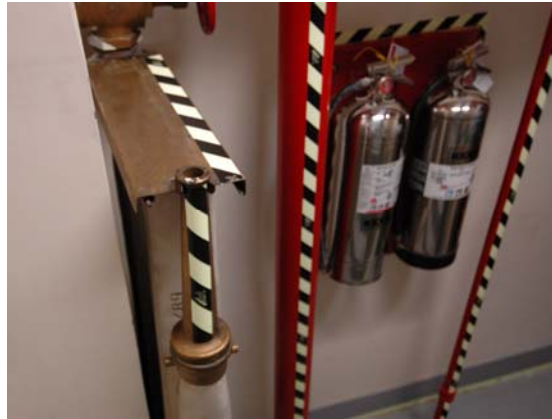
Exhibit 7 Obstacle tape installed.
