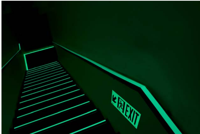
Exhibit 6 Photograph of an installation showing minimum compliance components for an RS 6-1 new building installation.
