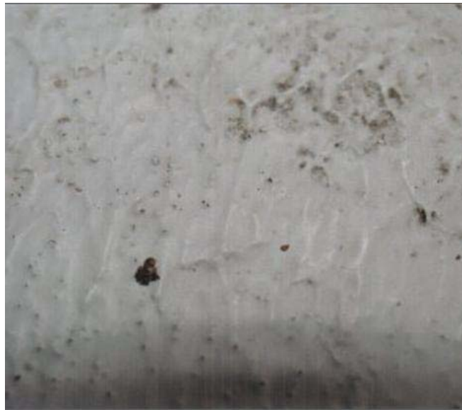
Figure 8. (A) Picture of the subject stairway. (B) Picture of the textured fiberglass landing surface containing imbedded abrasive non-skid particles.
