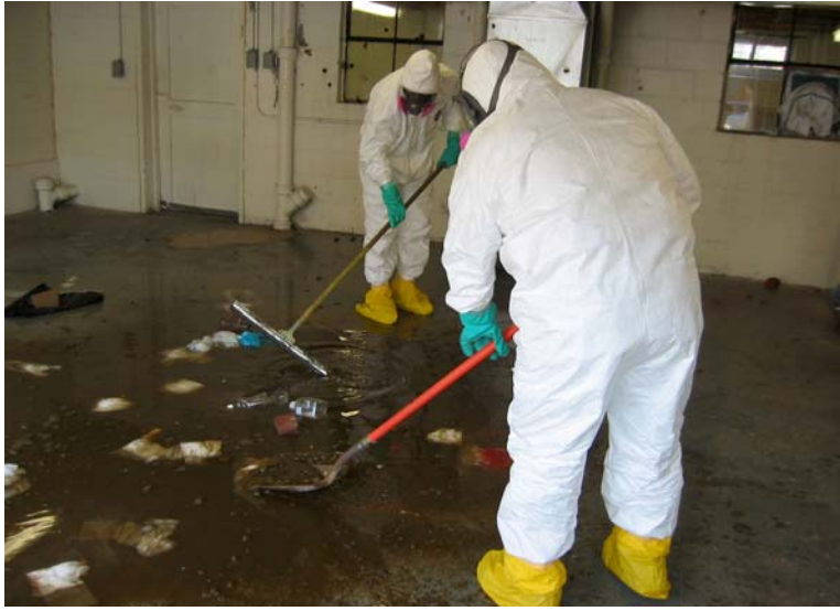
Exhibit 2. Workers removing flood residue wearing proper personal protective equipment.
