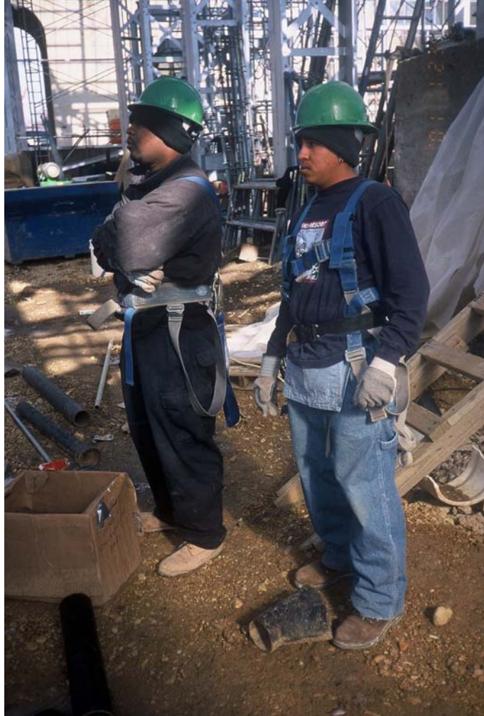
Exhibit 7: Proper Use of a Harness?
