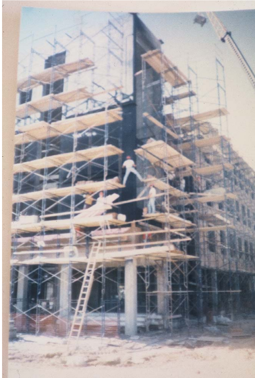
Exhibit 3: Foreman “Among the Missing”
