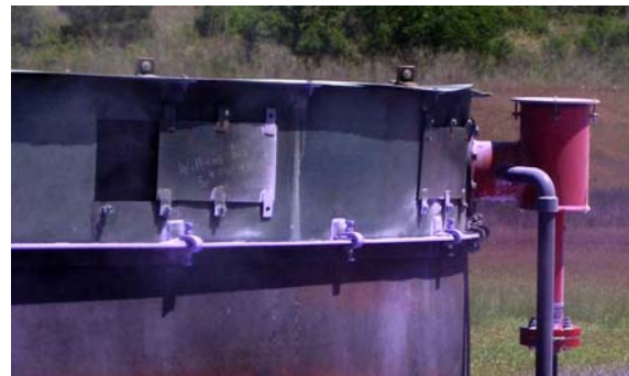
Exhibit 10 This foam chamber has dual agent capability,
