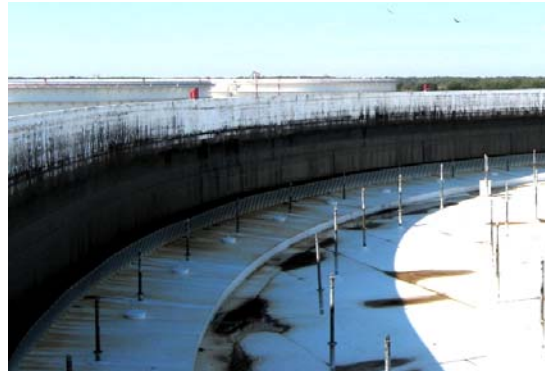
Exhibit 2. These pictures show external floating roof tanks from the ground and the top.
