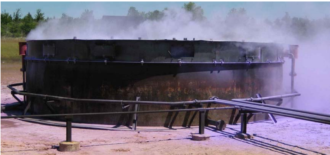
Exhibit 17 Dry chemical application following the foam extinguished residual appurtenance fires.
