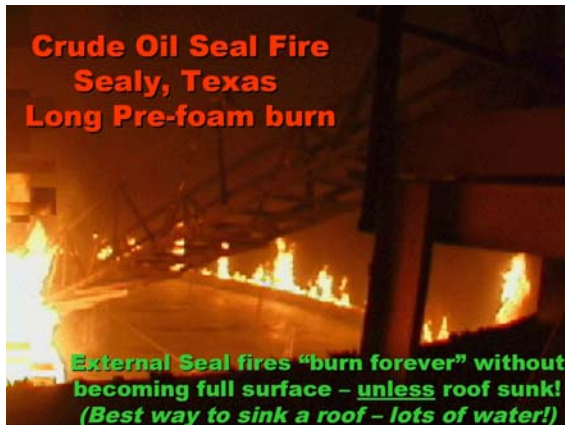
Exhibit 6. This Is an External Floating Roof Seal Fire.
