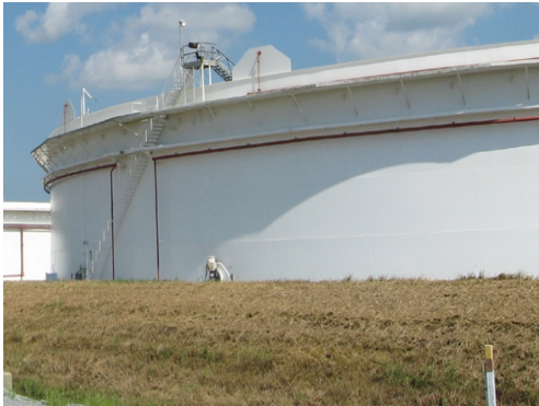
Exhibit 2. These pictures show external floating roof tanks from the ground and the top.
