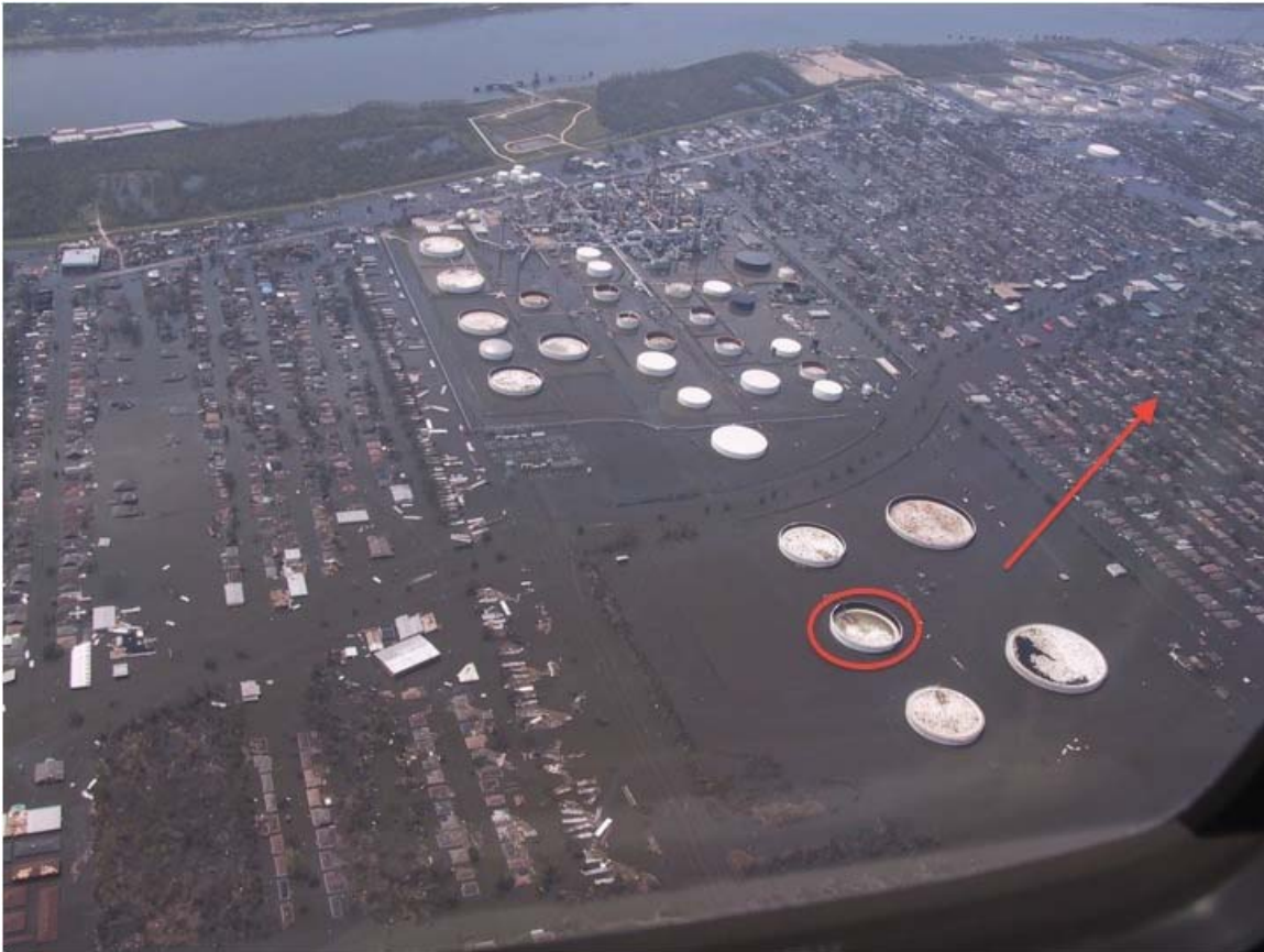
Exhibit 3. This photo from the 08/30/05 RNA flyover shows no oil from the damaged tank (red circle). The eventual direction of flow into Chalmette is shown by the red arrow.
