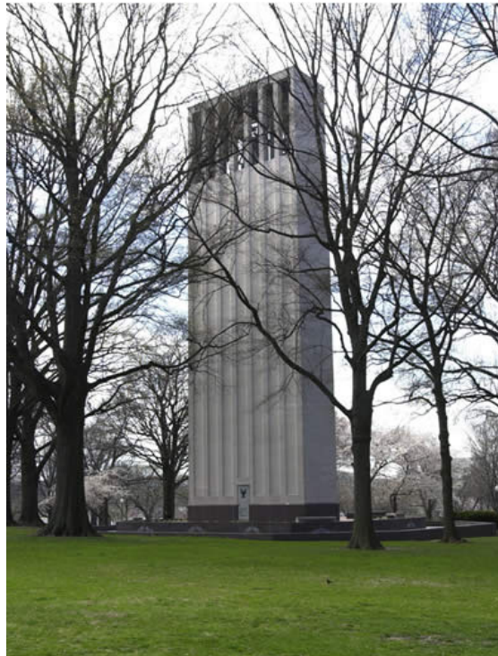
Exhibit 6: Using the PtD process eliminated fall hazards related to roof maintenance on the Taft Memorial.
