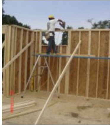
Exhibit 10. Framer working off of horse scaffold tying first floor walls together
