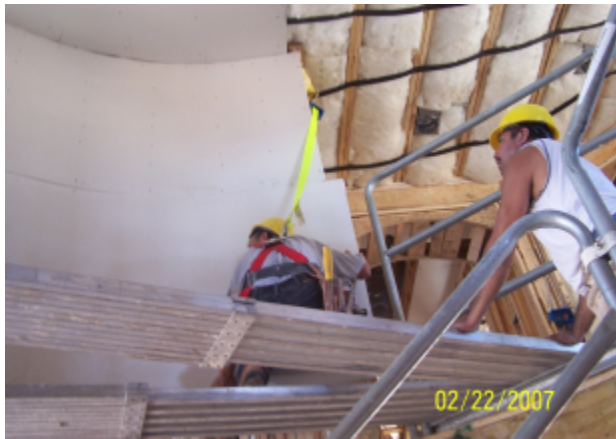
Exhibit 19. Dry wall hangers using PFAS with retractable lines in stairway area.
