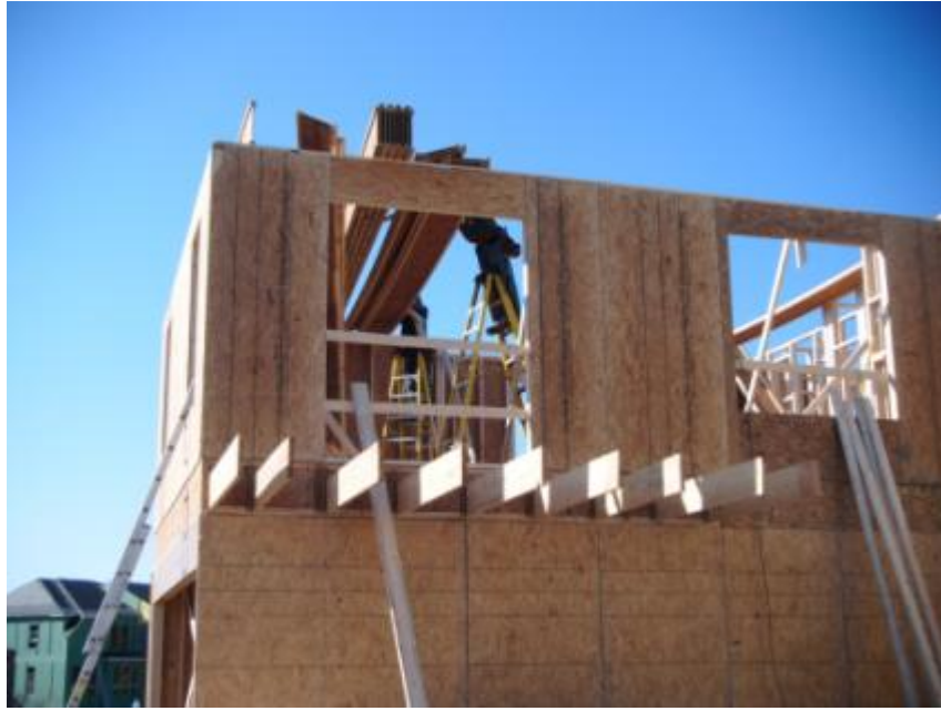
Exhibit 12. Framers installing second floor joists from ladders.
