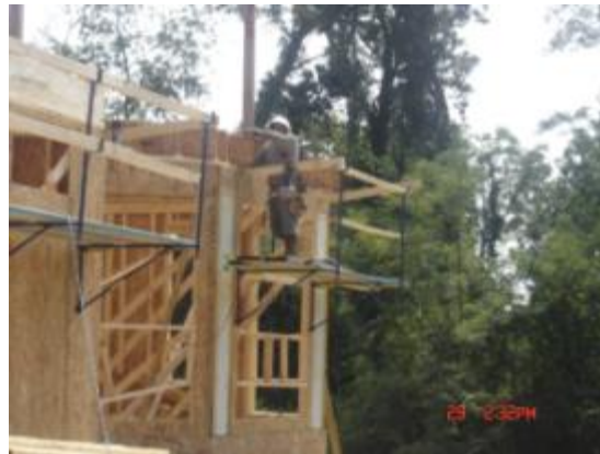
Exhibit 9. Framer working off of carpenter bracket scaffold installing second floor joists
