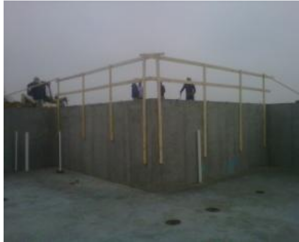
Exhibit 4. Guard rails installed on basement walls
