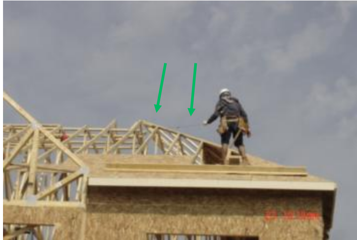
Exhibit 17. Worker sheathing roof using PFAS
