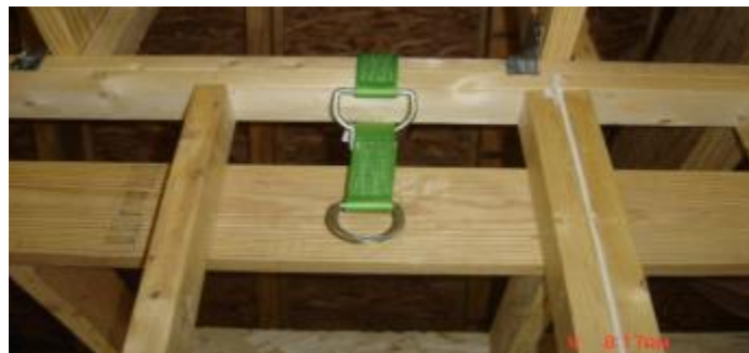
Exhibit 18. Anchor strap installed on double top plate of interior wall
