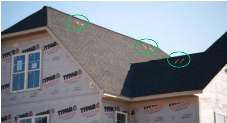
Exhibit 1. Permanent roof anchors installed for trades to use.
