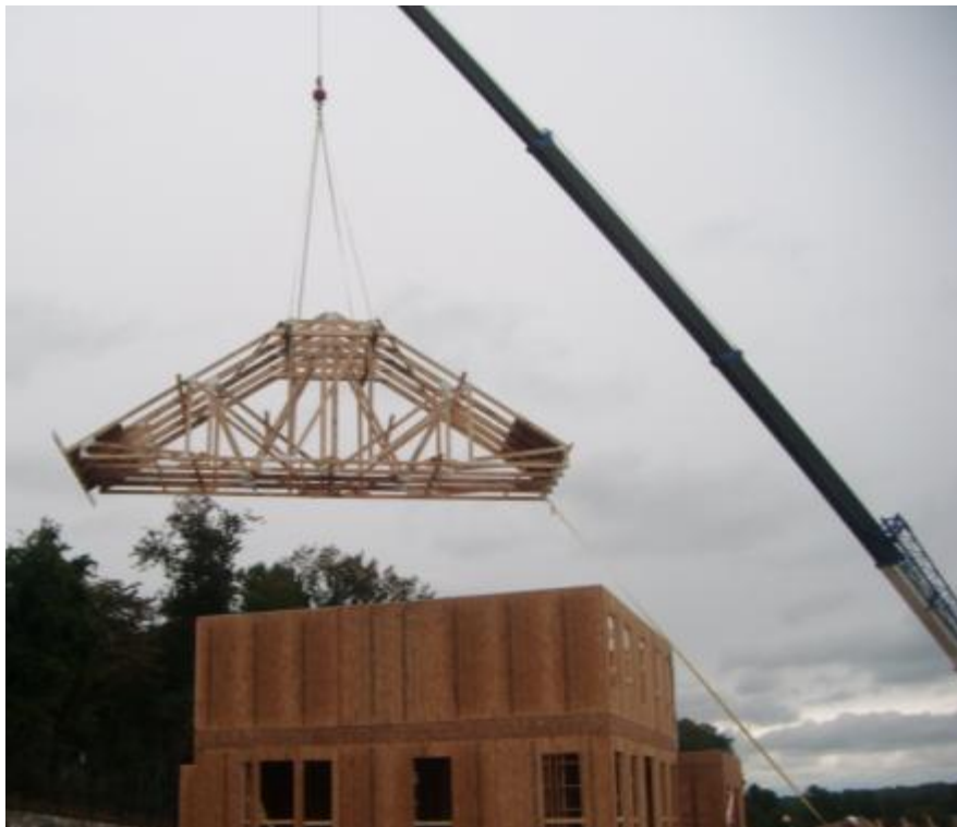
Exhibit 14. Braced trusses lifted by crane
