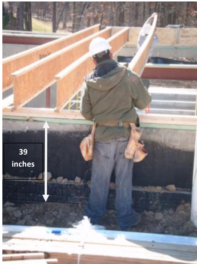
Exhibit 7. Framers installing floor joists from backfilled ground 39 inches from top of basement wall to ground and ladders
