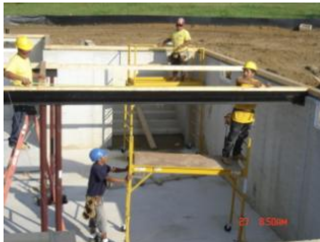
Exhibit 5. Workers setting sill plate on basement walls from ladders and mobile scaffold
