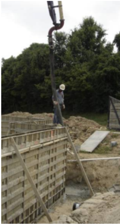
Exhibit 2. Concrete worker walking forms while pouring basement walls.
