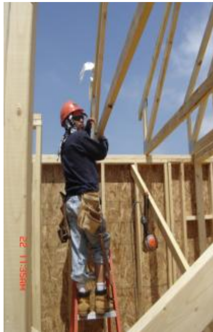
Exhibit 15. Worker working off of ladder while installing trusses.
