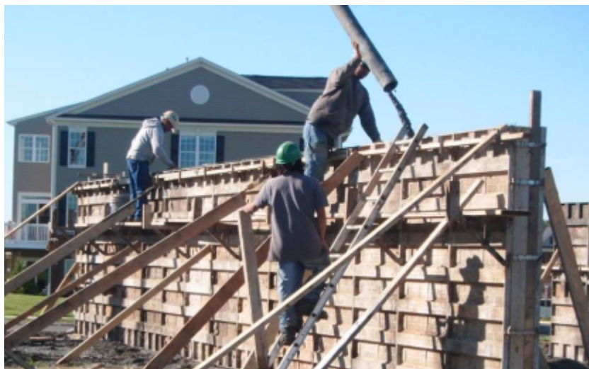
Exhibit 3. Concrete workers working off of bracket scaffold while pouring basement walls.
