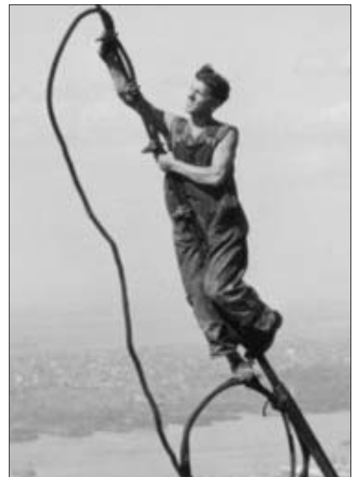
A worker strings cable—stories above the ground—on the Empire State Building construction site.
