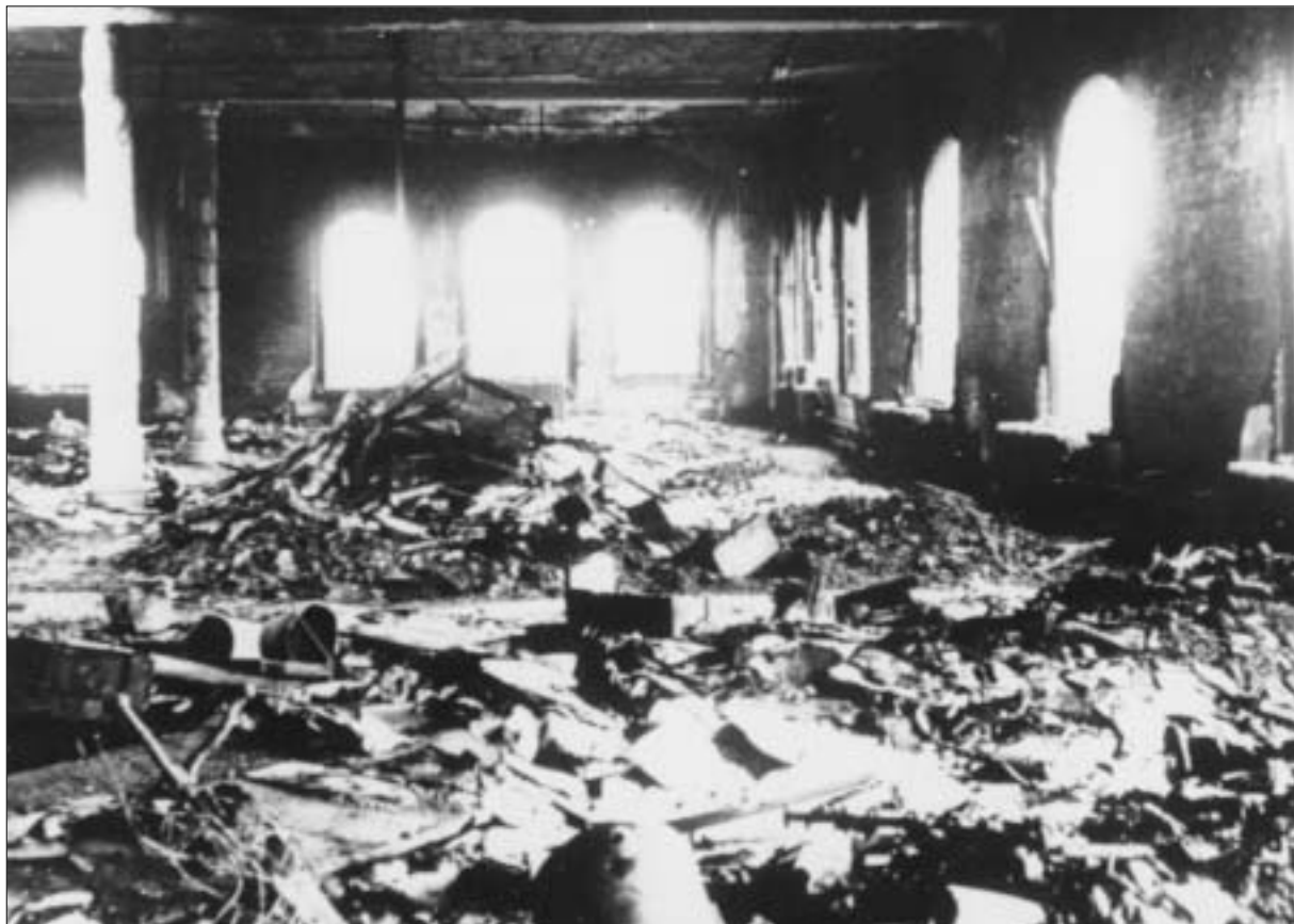
Tenth floor of the Asch Building, site of the Triangle Shirtwaist Co. fire in 1911.
