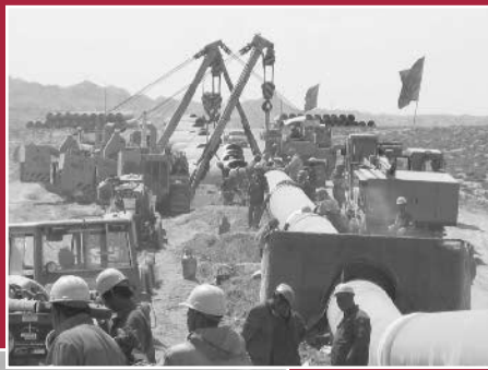
Photo 1 (top): WEPP construction site.
