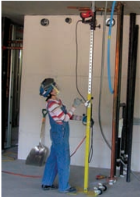
Photo 8 (above, left): A makeshift positive stop was added to prevent the drill bit from going too deep. The newer saddles have a built-in adjustable stop.
