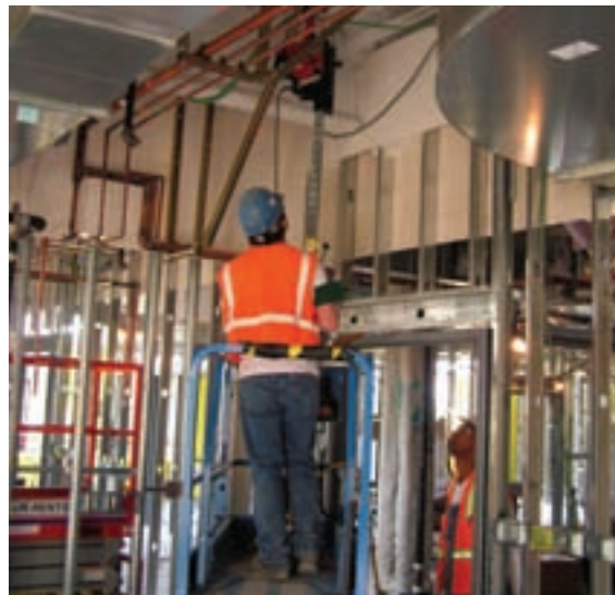
Photo 13 (above): The inverted drill press operated from a scissors lift. The clearance of the lift below the door header would require that the device be dismantled and removed in order to move the lift between rooms. Since the subjects had only two to four holes to drill per room, using the device for this application was inefficient and time consuming.
