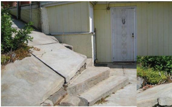
Photo 1: This stairway has high degree of variation in both riser heights and tread depths. If a riser is too high or too low, a person navigating the stairs may find it difficult to maintain safe footing. Treads that are too short force the stair user to either rest only part of a foot on each tread or to twist the foot unnaturally.
