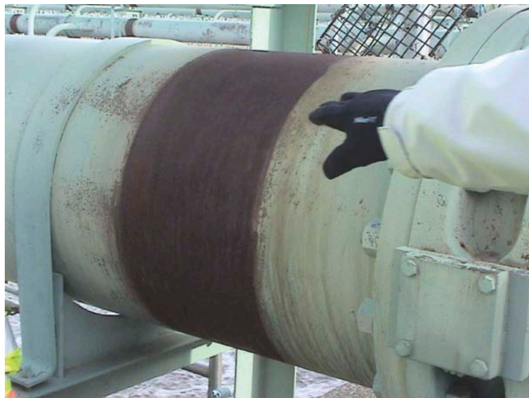
Pipe with lead-containing paint removed to facilitate torch cutting.
