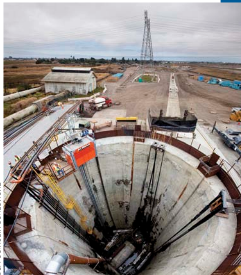
Photo 3: Water System Improvement Program (WSIP) Bay Tunnel shaft.
