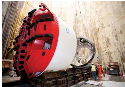
Photo 2: Tunnel boring machine (TBM) cutter in the Bay Tunnel.
