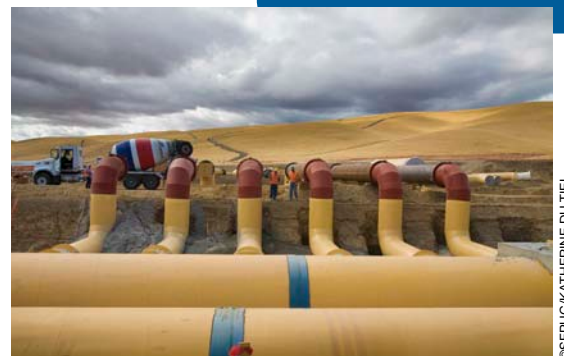
Photo 6: WSIP Tesla UV treatment piping.
