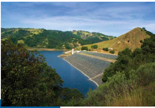
Photo 7: WSIP Calaveras Dam preretro.
