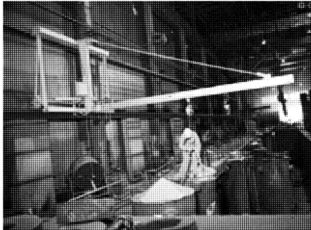
Figure 20. Swing arm allows area coverage and eliminates swing falls
