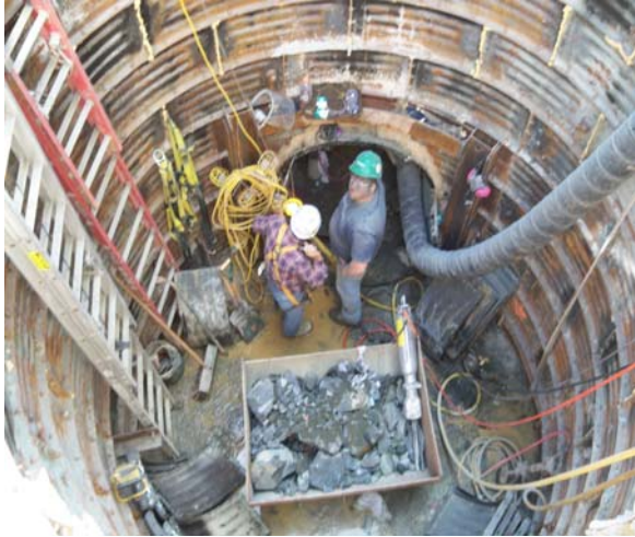
Exhibit 5. Hard rock shaft and tunnel.
