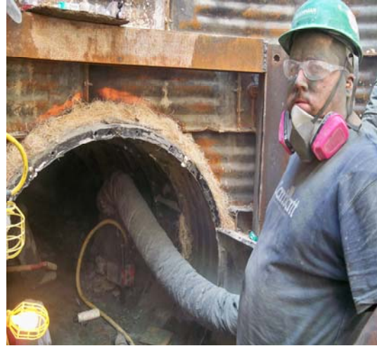
Exhibit 6. Ventilation and PPE.
