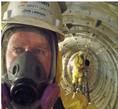
Exhibit 1. Permit-required confine space entry.
