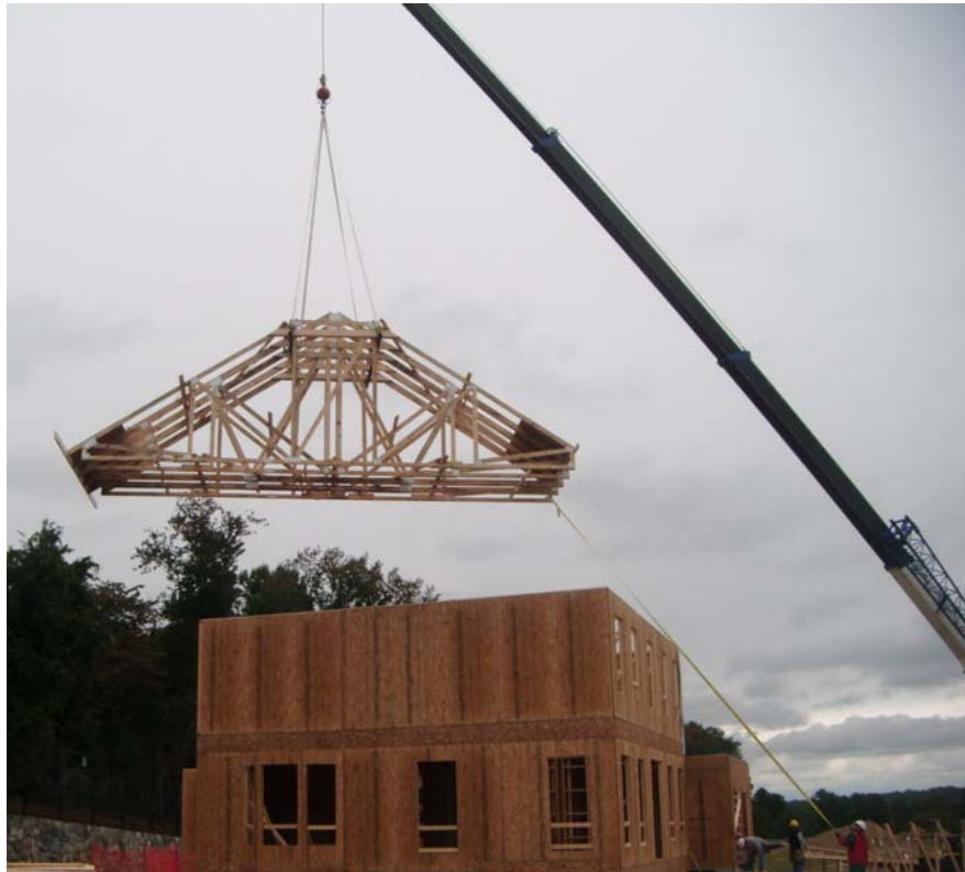
Exhibit 14. Braced trusses lifted by crane.
