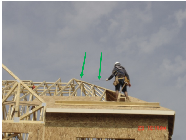
Exhibit 17. Worker sheathing roof using PFAS.
