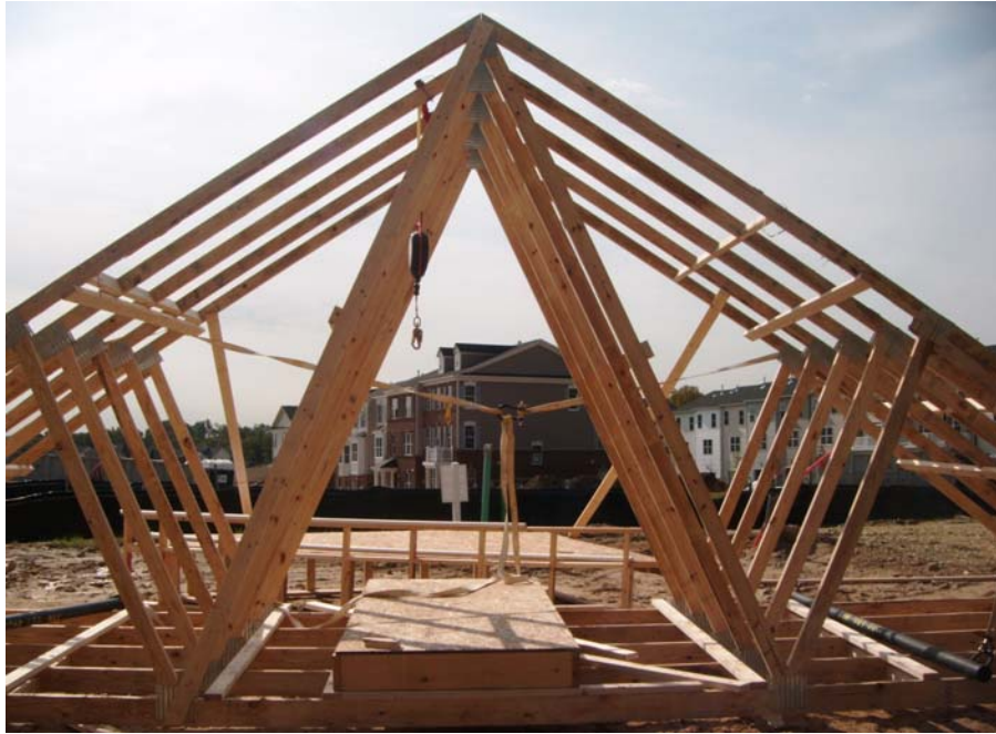
Exhibit 13. Braced trusses with temporary anchor point installed and self-retracting line.
