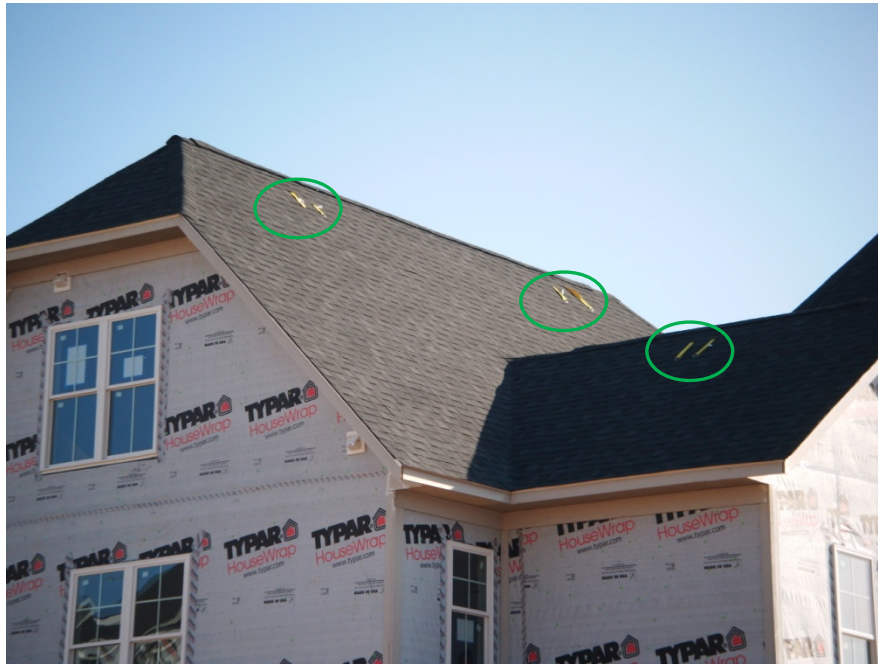
Exhibit 1. Permanent roof anchors installed for trades to use.
