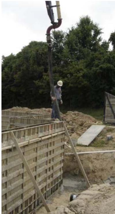
Exhibit 3. Concrete worker walking forms while pouring basement walls.
