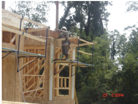
Exhibit 9. Framers working off of carpenter bracket scaffold installing second floor joists.
