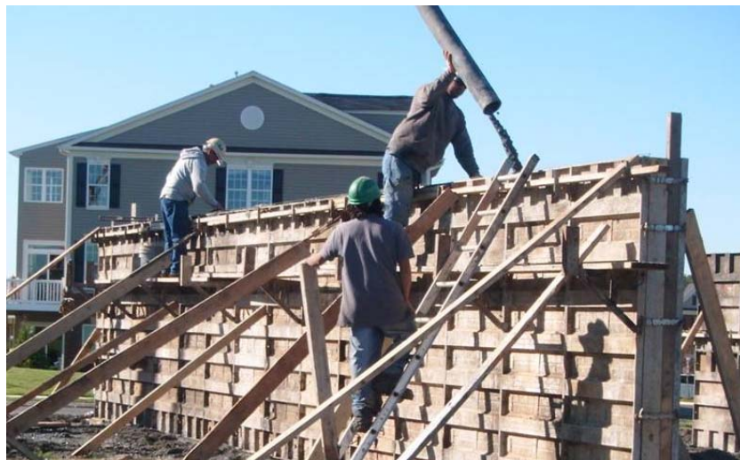
Exhibit 4. Concrete workers working off of bracket scaffold while pouring basement walls.
