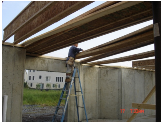
Exhibit 6. Framer working off of a ladder installing first floor joists.
