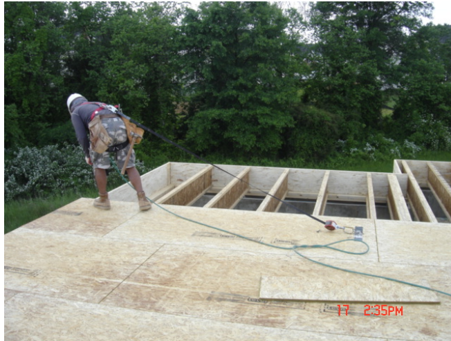
Exhibit 8. Worker using PFAS during installation of floor sheathing.
