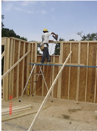
Exhibit 10. Framers working off of horse scaffold tying first floor walls together.
