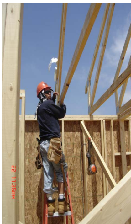
Exhibit 15. Worker working off of ladder while installing trusses.
