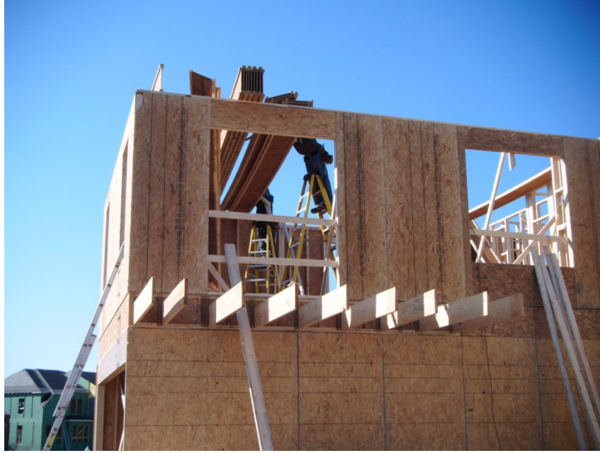
Exhibit 12. Framers installing second floor joists from ladders.
