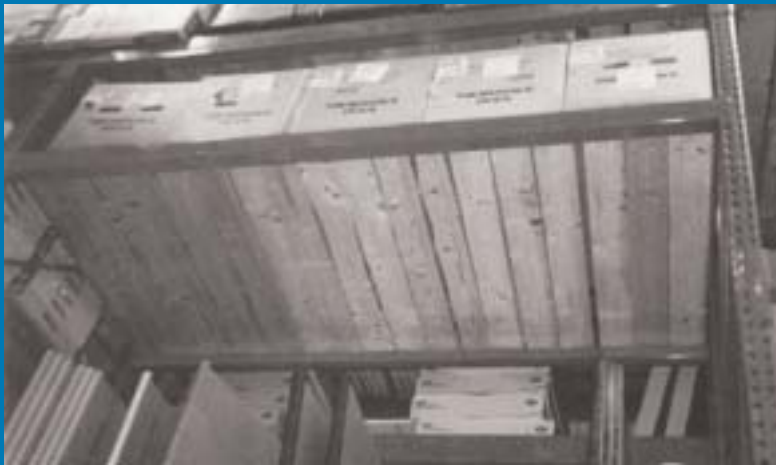
Photo #8 (above) shows loose wooden planks placed in between the cross-members.
