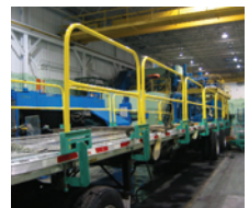
Photo 9: Temporary guardrails are a measure that can reduce falls from the trailer.
