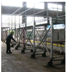
Photo 7: A roll-up catwalk provides safer access during tarping.
