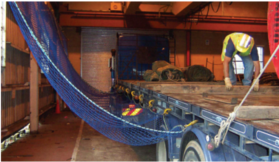
Photo 10 (above): A fall arrest net system can be attached to the flatbed frame to form a trough to fall into on either side of the trailer.
