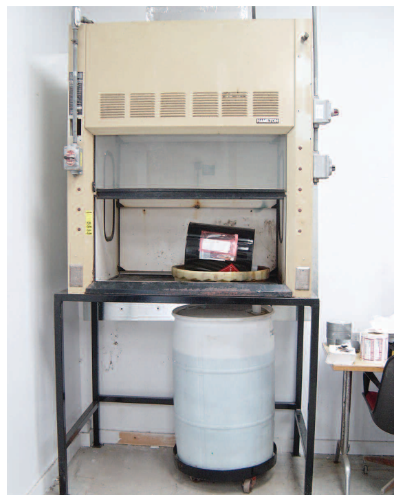
Photo 2: EHRM staff modified a fume hood at the hazardous waste facility, which allowed for more bulking with a higher comfort level for EHRM waste personnel.
