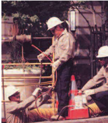
Protective clothing rated for thermal protection from arc flash hazards ranges from shirt and pants uniforms (as shown) to switching suits and head protection for higher thermal energy exposures. (Photo courtesy of DuPont)
