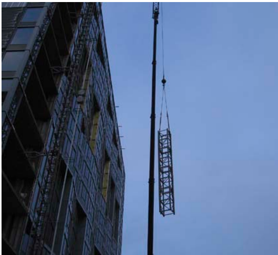
Photo 2 (top, left). Ironworkers installing the hoist mast sections in place with 100% tie-off. Photo 3 (top, right). A city street blocked off during a hoist dismantle operation. Photo 4 (above). Hoist mast dismantle in progress with an assist mobile crane.
