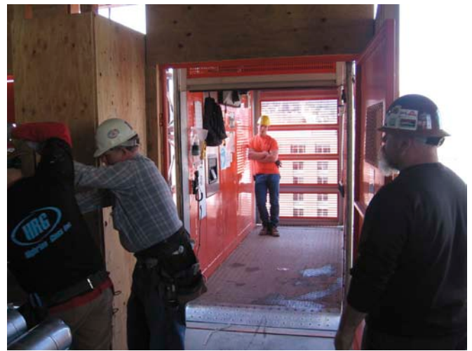
Photo 5 (left). Construction hoist with hoistway protection on each floor. Photo 6 (right). Operators should maintain clear path during loading operations.
