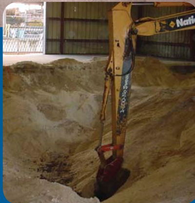
Photo 5: Source removal for remediation occurred inside a warehouse building for this project. The structural integrity of the building and air quality monitoring (for heavy machinery exhaust) were evaluated as part of this site's safety and health program.
