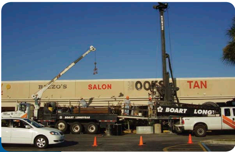
Photo 2: During sonic drilling, a large work area is needed for support vehicles. The work area required for different drilling methods is an important safety and health consideration for work at a facility or property.
