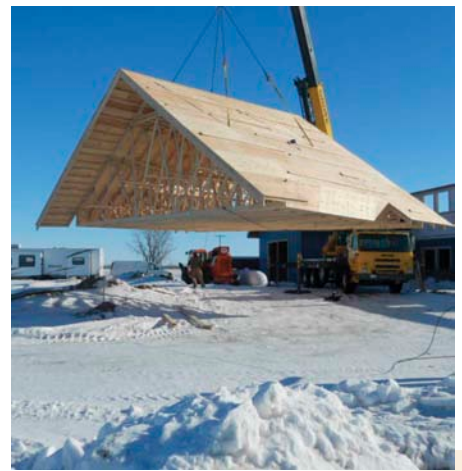
A roof built on the ground (Photo 5) being placed on a structure.
