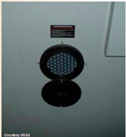
From top: A simple device (Photo 9) allows the safe insertion and removal of breakers while the installer is a safe distance away. Viewing ports (Photo 10) allow for inspection and measurement from outside the panel.
