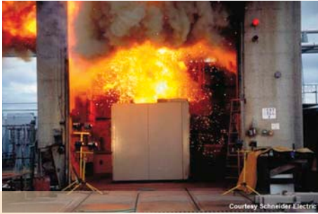
In Photo 8, an arc-rated switchgear test shows arc-flash energy channeled away from where a person could be standing.
