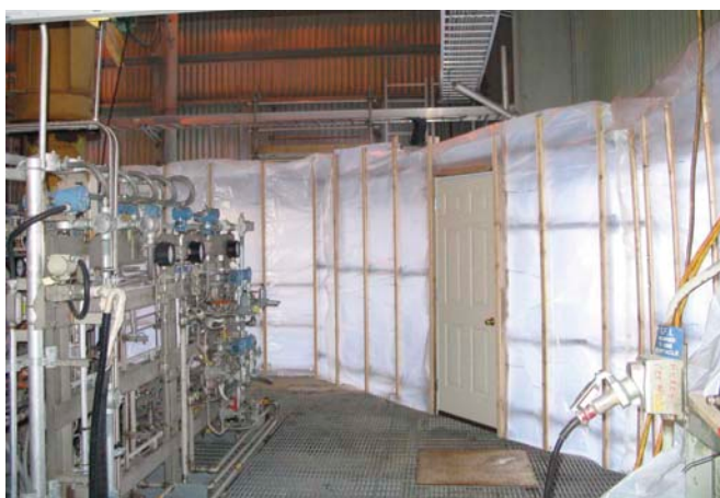
Photo 3 (above): Congestions and confinement created by equipment/buildings.
