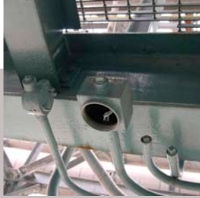
Photos 9 and 10: Routes of entry for flammable vapors and gases into electrical conduit.
