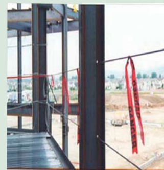
(Clockwise from top): Photo 9 shows industrial stairs, which are preferred to access a work platform, mezzanine, upper level or roof. Photo 10 depicts why specifying holes in columns at 21 and 42 in. above the floor slab makes it easy to install cable or wire perimeter cables. Photo 11 shows the value of depicting rebar details on design drawings.
