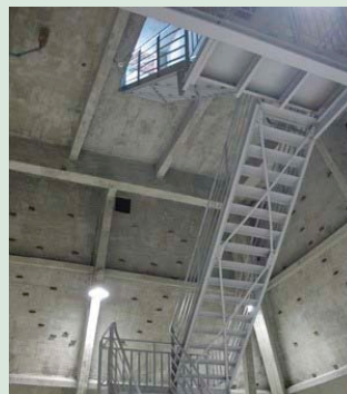
(Clockwise from top): Photo 9 shows industrial stairs, which are preferred to access a work platform, mezzanine, upper level or roof. Photo 10 depicts why specifying holes in columns at 21 and 42 in. above the floor slab makes it easy to install cable or wire perimeter cables. Photo 11 shows the value of depicting rebar details on design drawings.
