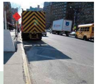
Photo 5 shows shadow vehicles, which provide notice to approaching traffic and physical protection to workers.
