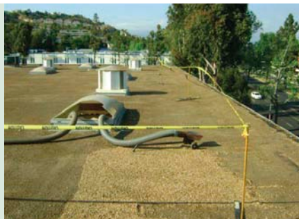
Photo 7 was taken after a fall through an unguarded skylight.
