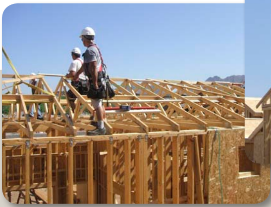
(Clockwise from top left) Photo 1: Workers protected from internal swing fall hazards, within the 30° arch due to minor additional bracing, and outside 30° where the force of gravity is cancelled due to the friction of the cable against the incline of the trusses.
