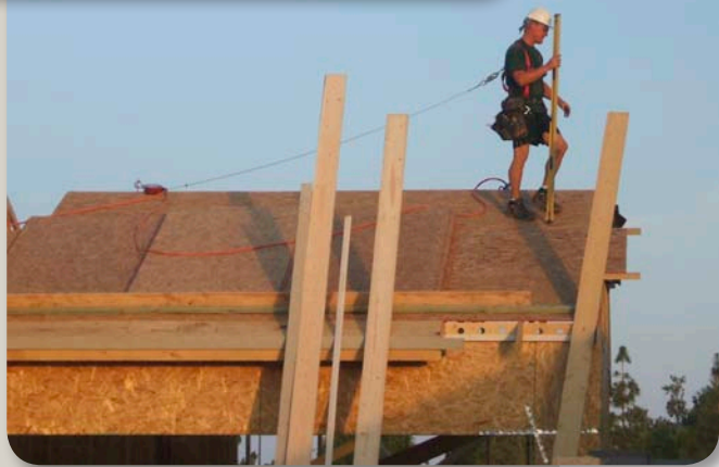
(Clockwise from top left) Photo 1: Workers protected from internal swing fall hazards, within the 30° arch due to minor additional bracing, and outside 30° where the force of gravity is cancelled due to the friction of the cable against the incline of the trusses.
