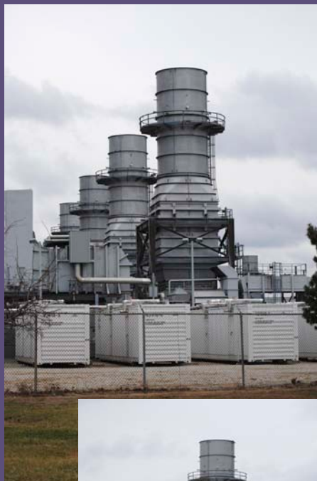
Photos 1 and 2: Examples of peaker units. Peaking power plants, also known as peakers , are power plants that generally run only when there is a high (peak) demand for electricity.
