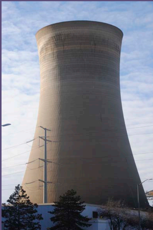
Photo 8: Cooling towers may harbor Legionella; activities to maintain cooling tower pumps, inspect and service equipment, collect samples, clean screens or add chemicals to circulating water systems may expose workers.
