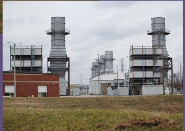
Photos 1 and 2: Examples of peaker units. Peaking power plants, also known as peakers , are power plants that generally run only when there is a high (peak) demand for electricity.
